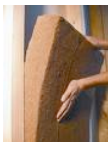
Cellulose (left) and wood fibre (right) being installed
