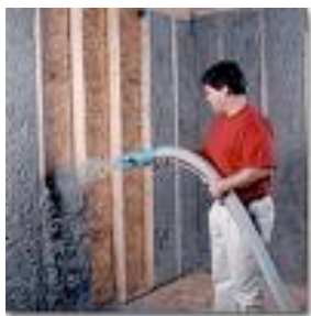
Cellulose (left) and wood fibre (right) being installed
