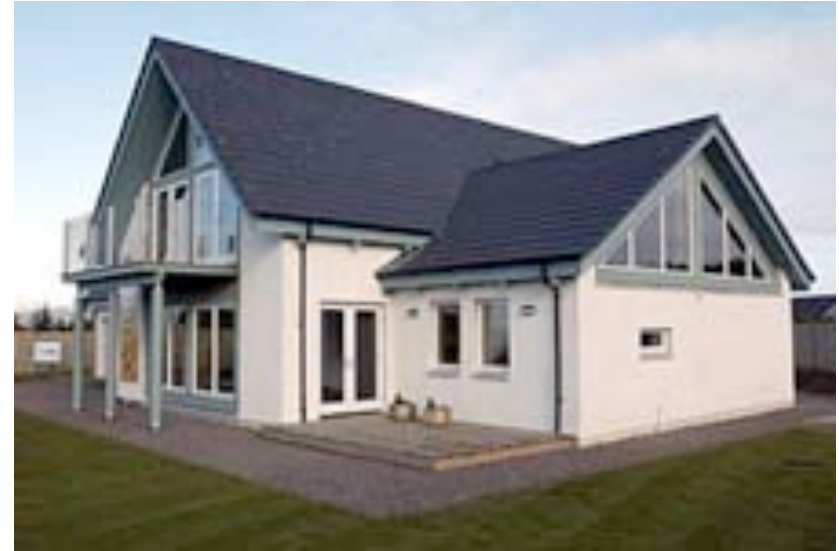
The south-facing Super E house
