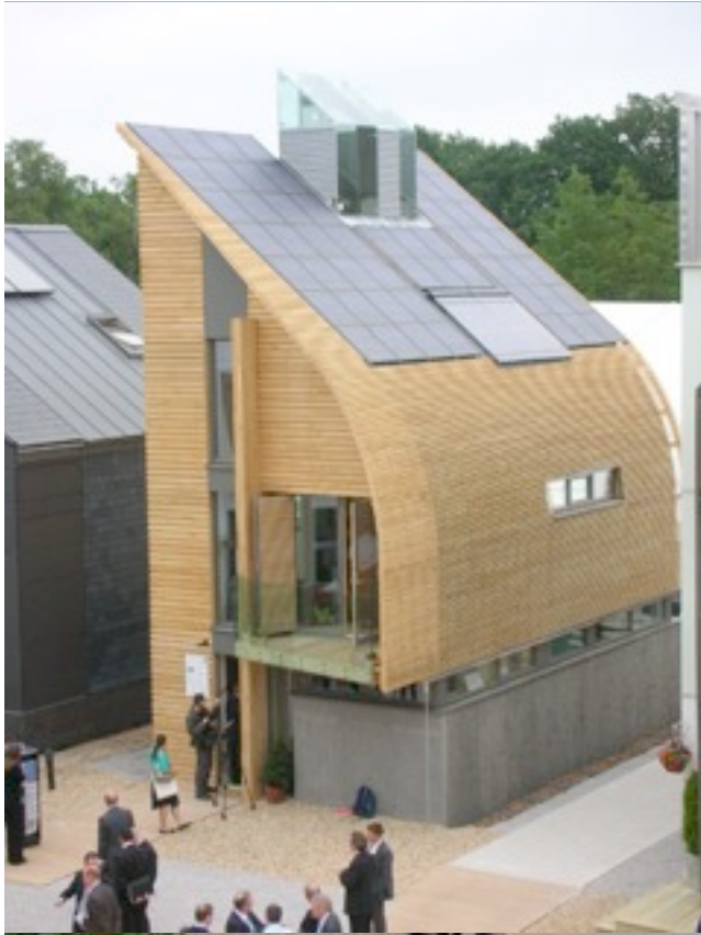
The north-facing Kingspan Lighthouse
